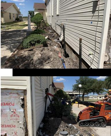
Heavy rains during the spring and early summer of 2021 delayed the start of this project. When the weather finally cooperated, Ram Jack crews were able to install the required helical piles and raise the exterior beam 12 to 15 inches.
