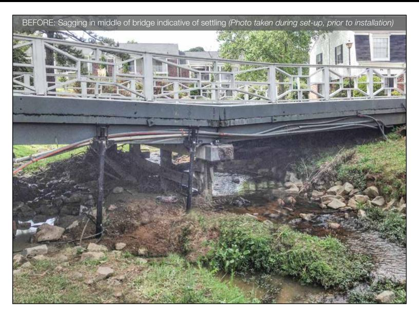
A bridge supported by driven wood piles, connecting two sections of an apartment complex designed for vehicles, crosses a 20 ft. wide creek. The fire marshal had been monitoring the bridge for several years to ensure emergency vehicles could use the bridge safely. The settlement of the bridge was deemed unsafe; if the bridge wasn't repaired, the apartments would be condemned.
