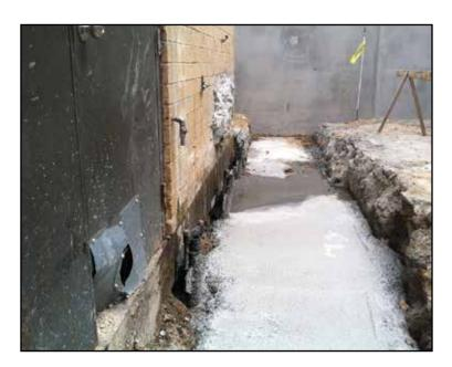
During installation of the piles, the Ram Jack crew ran into a number of issues, having to make their way around concrete as well as drive one of the piles to a depth of 35 ft. After some significant excavation and diligent work by the crew, the driven piles were successfully installed, and the building's structural integrity was restored.
