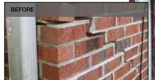
stabilize the corner of the home and lift the sagging structure. Due to shallow footings, low profile brackets would be needed to prevent the repair materials from being visible after the repair was complete.
