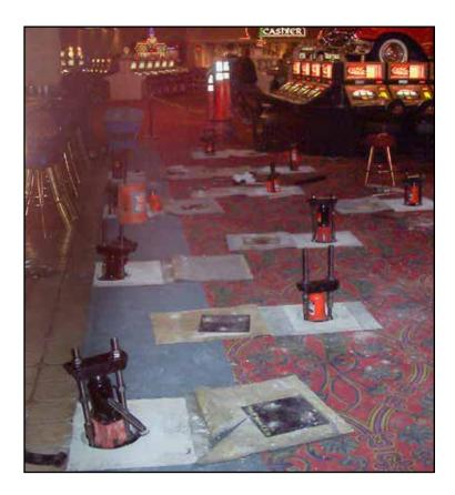
elevation. A Ram Jack retaining system was used to tighten and hold the slab in place. After the jacking system was removed from all holes, a line pump injected sand slurry under the slab to fill any voids, and all of the cored holes were filled. The engineers and maintenance workers at the SLS Hotel and Casino were more than impressed with the quality work performed by Ram Jack Las Vegas as well as the fact that the job was done with minimal interruption to casino business.
