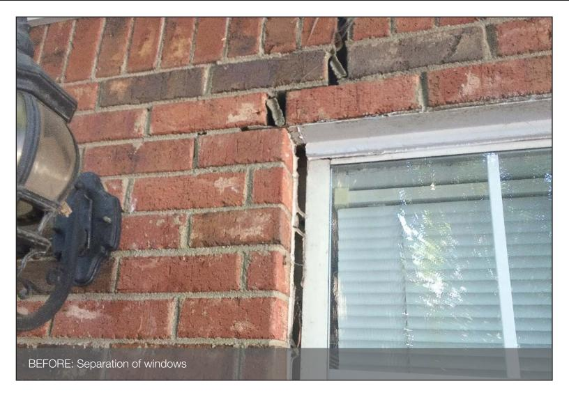
A telltale sign of foundation damage is separation of windows, floors, and doors from the walls to which they were originally tightly connected. As the foundation settles, the walls come with it, causing gaps to form or windows and doors to fit improperly. This might translate to unwanted drafts coming through newly formed openings or for windows and doors to no longer open and close properly.
