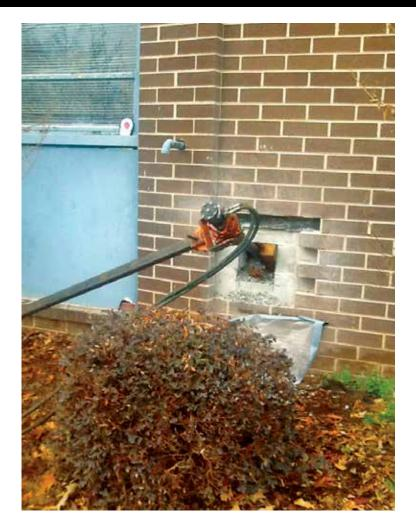
Helical tie-back anchors with threaded connections permanently stabilize leaning exterior walls
