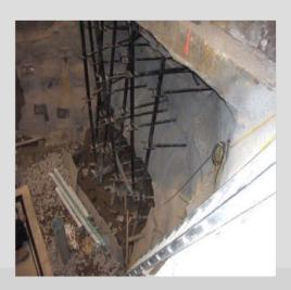
**Situation:** The project consisted of an existing manufacturing facility requiring the installation of a 25'-0 deep precast concrete pit on the interior of the building. The opening of the excavation through the floor slab was approximately 30'-0 x 30'-0 and adjacent to a building column supporting a 133 kip load. Another obstacle encountered was the water table was 12'-0 below finished floor requiring the dewatering of the lower 13'-0 of the excavation.
